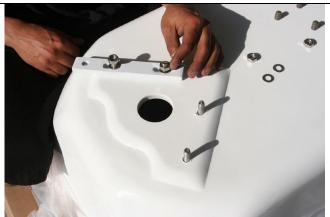
4. Place the claw foot in position. Hold the claw foot in position against the tub as you screw in the foot fixing bolt.
