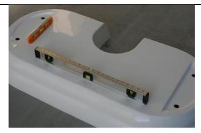
3. Make fine adjustments to the adjustable legs to ensure all four connect to the floor to make the tub base stable.
