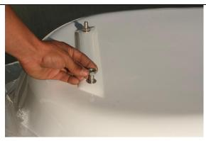
7. Place the pedestal onto the tub and attach it to the tub using the nuts and washers just removed.
