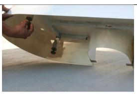
4. Mark off the holes for fixing the tub base to the floor.
