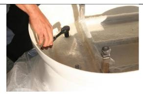
8. Turn the tub upright and position it over the drilled fixing holes. Use a screw or bolt to suit your floor material.
